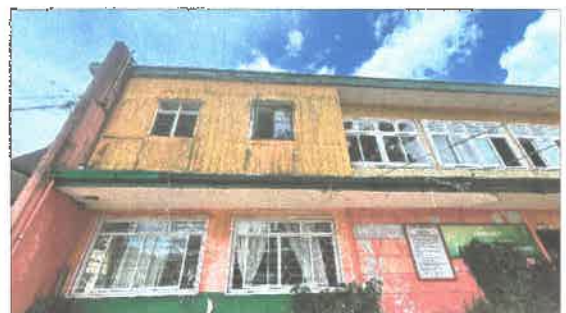
Existing UBA Office windows without canopy ( above)
